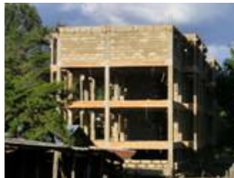
Staff flats walls going up!!
