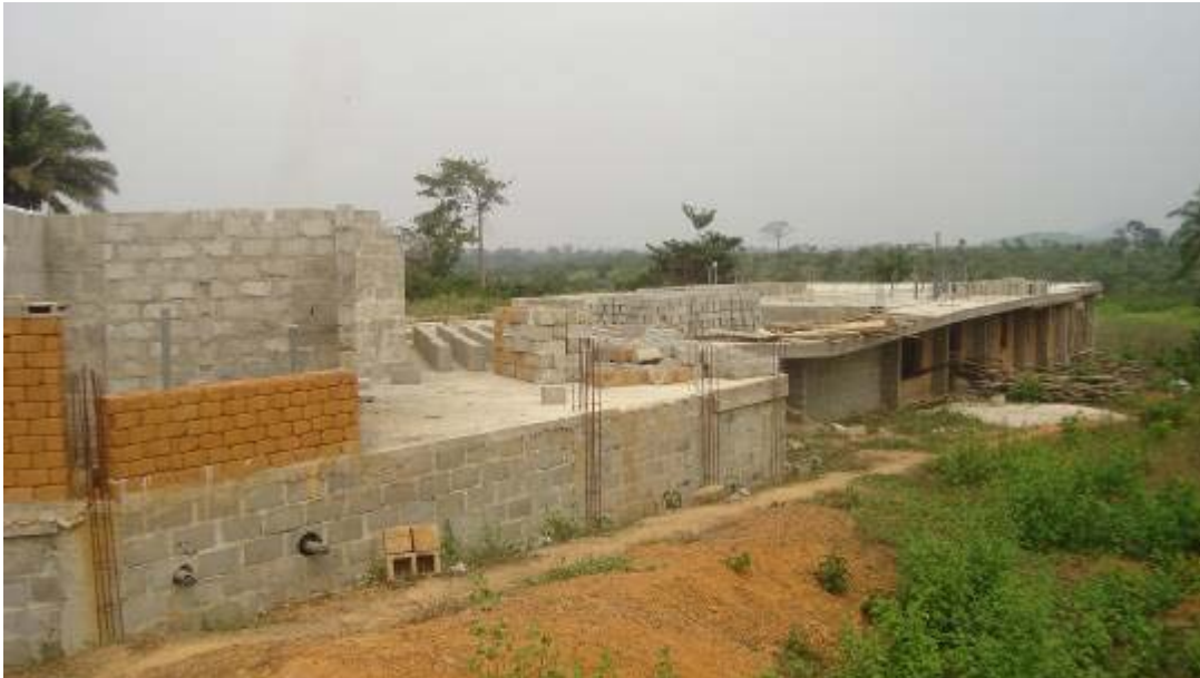
DENTAL UNIT JOINING THE MAIN LOBBY
