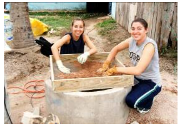
Alyson Waeltz & Melissa Swanson prepare mezccla, the solid components of mortar
