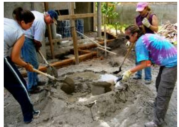
Mixing mortar takes teamwork
