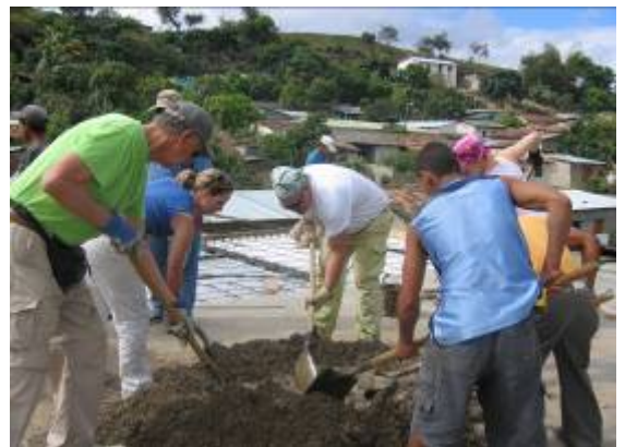
Mixing and Pouring Concrete during Week 2 Construction
