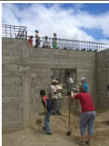
Construction on the Church Building during Week 1
