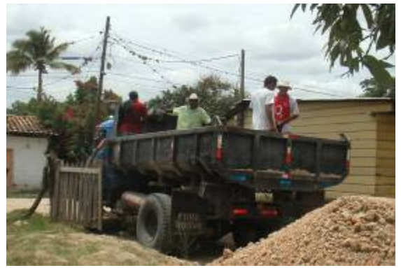
Delivery of “material select” to level area around the parsonage
