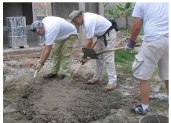
Hand mixing cement is back breaking work
