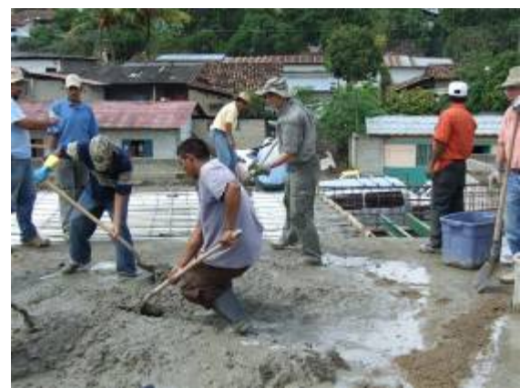
Time Honored Hand-mixing of Concrete
