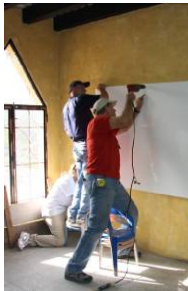
Installing a new “white board”
