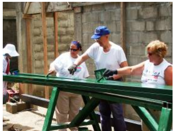
Painting Beams prior to Installation
