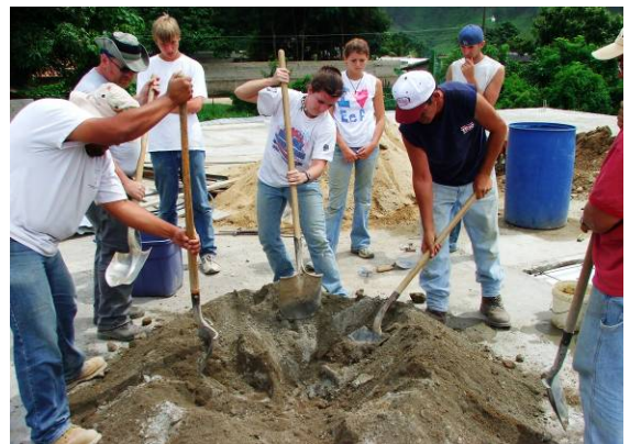
Mixing Concrete in the Time-Honored Way
