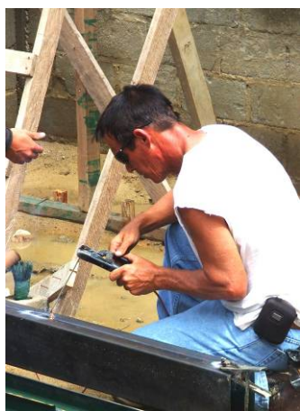
Jon Welds Beams – “Hot Work”
