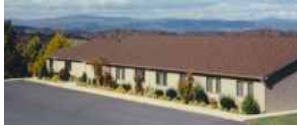
Blessings Lodge at Camp Overlook
